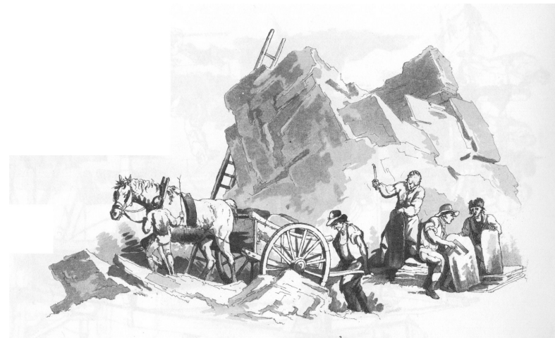
Irish navvies breaking up the rock into blocks for use in the cut masonry walls.
